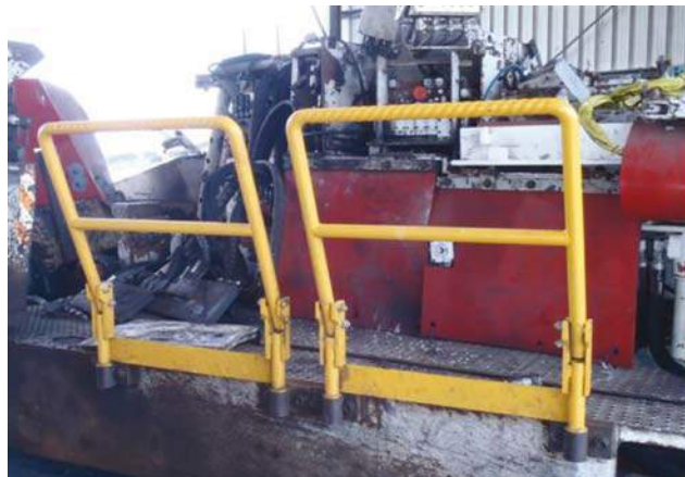
Continuous Miner Hand Rail Project - QLD
